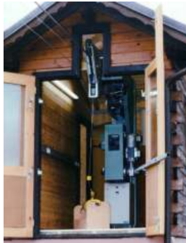
SEBA cable way installation with electrical double drum winch SDW-E
